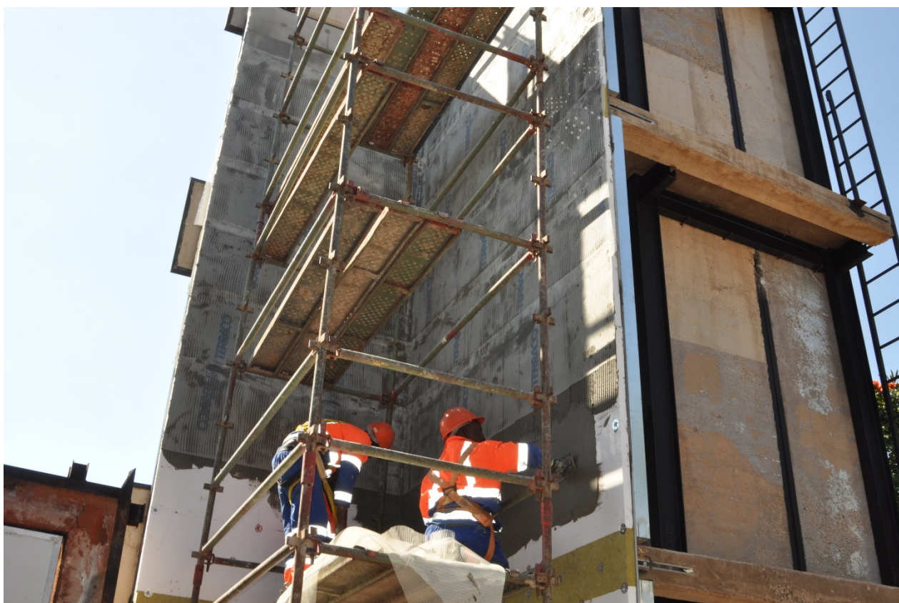
Mesh applied to the EPS and StoneWool
