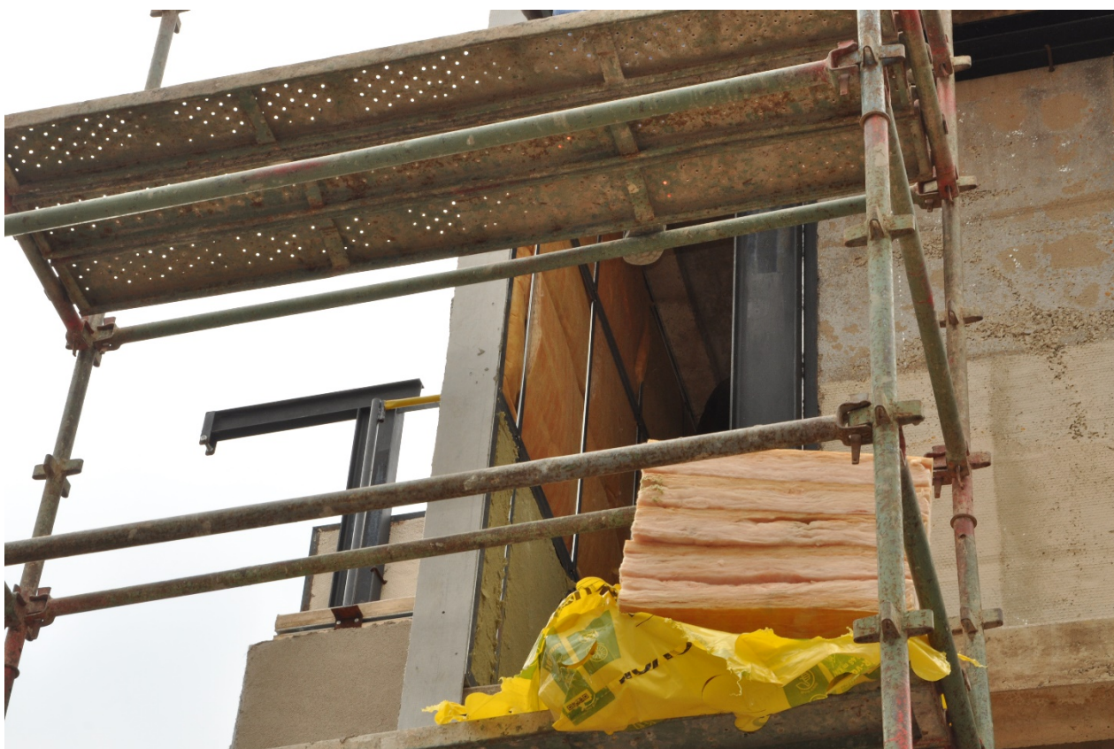
StoneWool and CavityBatt inserted in to the frame
