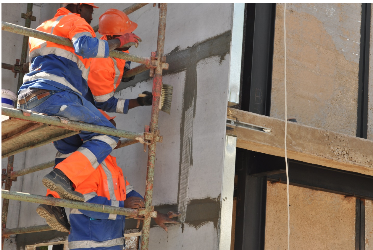
Coat and mesh applied to the joints of boards
