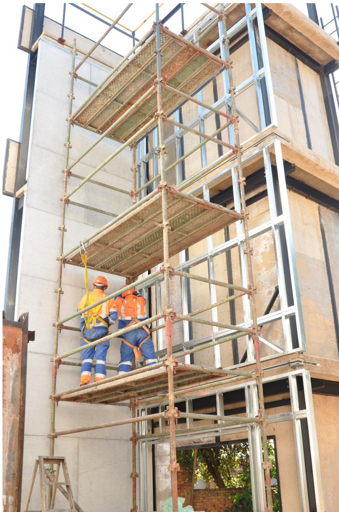
Steel frame anchored and MgO boards fixed to the frame
