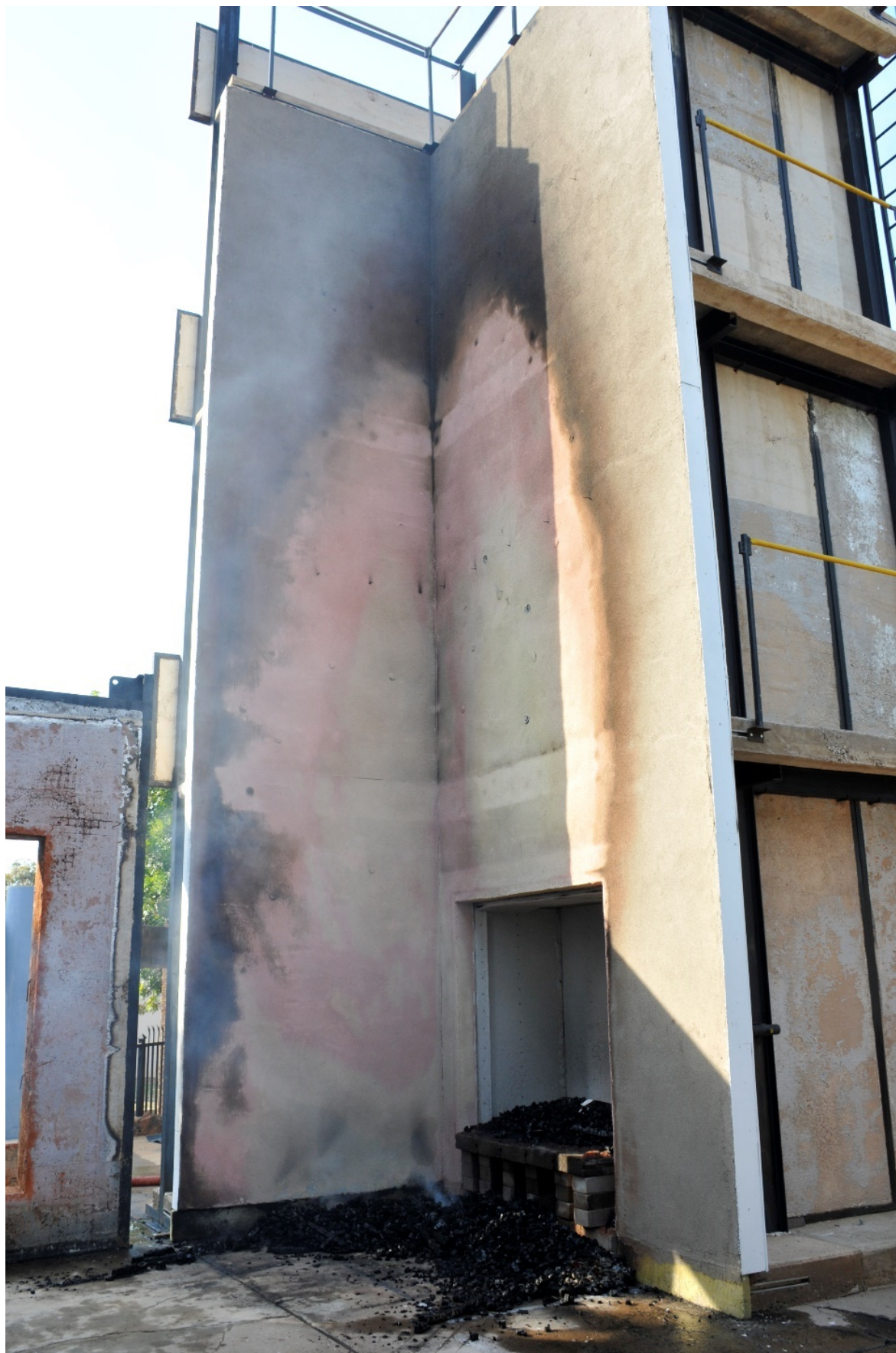
Figure 3.18: Specimen at conclusion of the test
