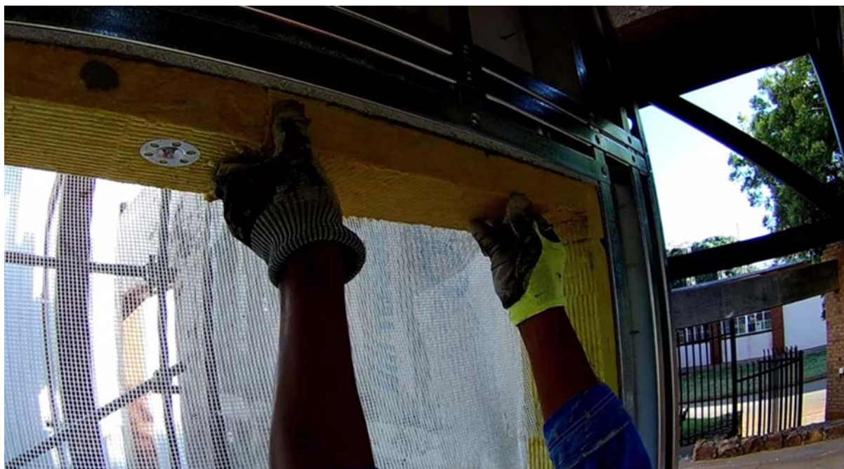
StoneWool applied in the Combustion Chamber
